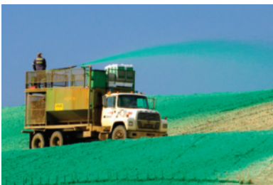
Figure 11 Special mixtures containing grass seeds may be sprayed on areas vulnerable to erosion.
