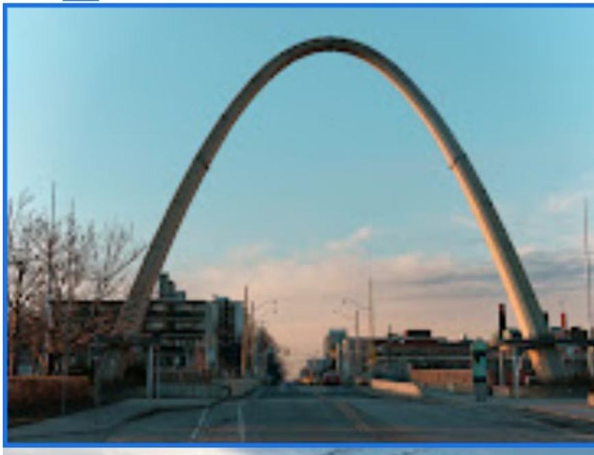
The Dufferin Gate is a parabolic arch that is approximately 20 meters tall and approximately 22 meters wide.
